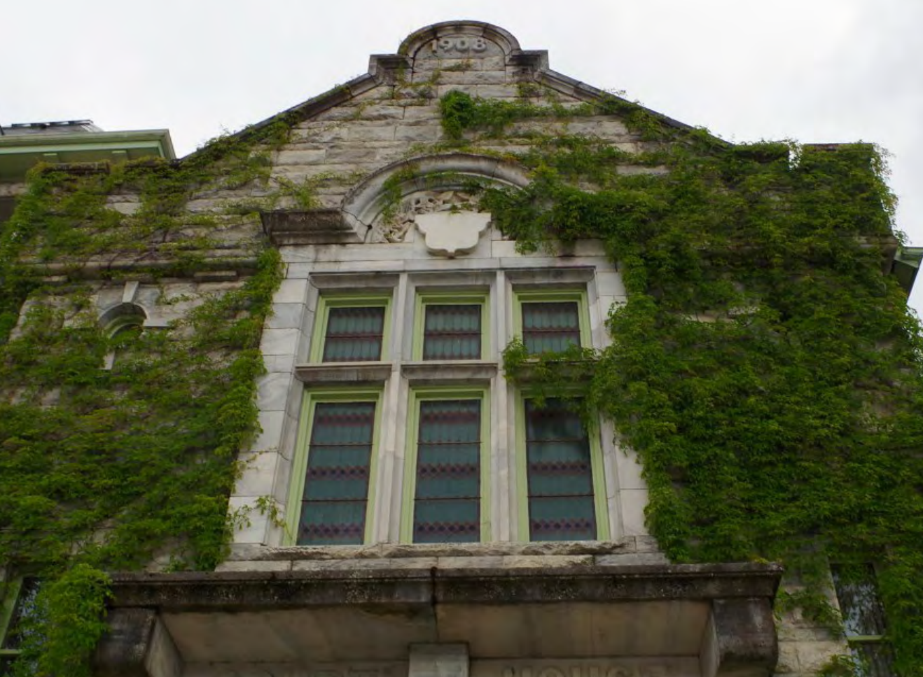
Nelson Courthouse | Credit: John Deacon, KC
